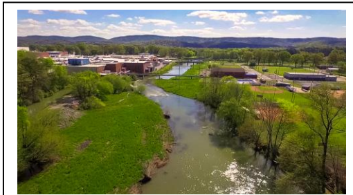
Mount Vernon Mills on the banks of the Chattooga River in Trion, Georgia. Photo from upstream at the Chattooga Dam.
